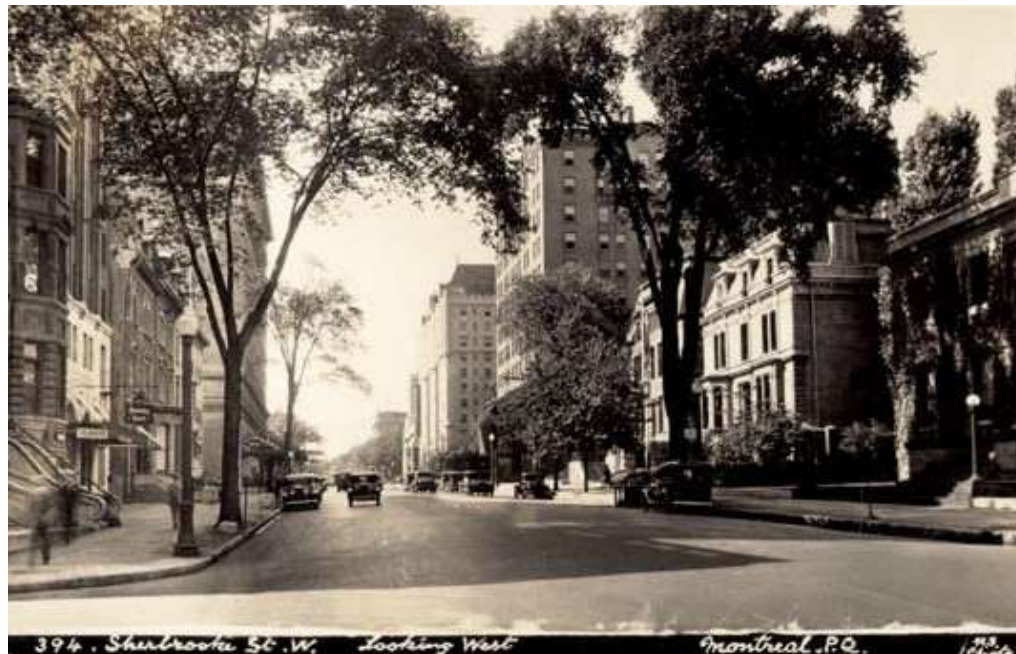
● Postcard of Sherbrooke Street, about 1934. On the right hand side of the photo, the Forget house is immediately to the right of the tree.
